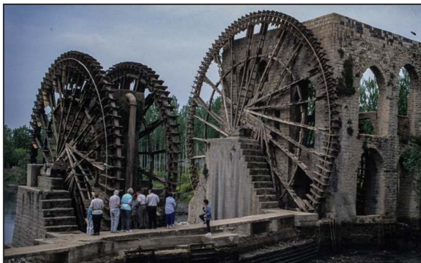
Noria waterwheels at Hama, which raised water onto the stone aqueduct.
